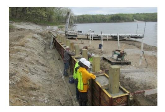
The students also constructed an ADA-accessible concrete sidewalk to replace the gravel at the edge of the lake.
